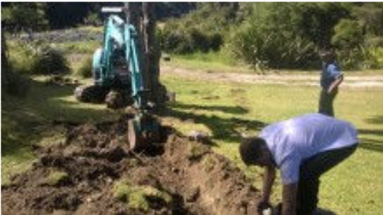
Laying grey water drainage from self contained cabin
